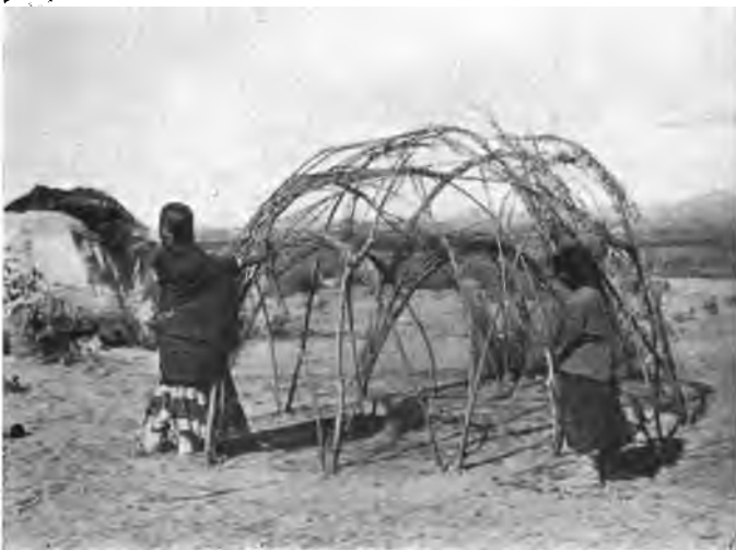
San Carlos Apache Women building a House.
